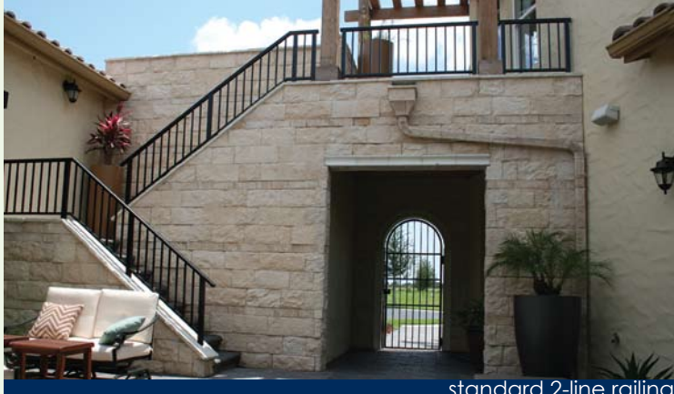
standard 2-line railing
