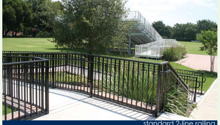
standard 2-line railing
