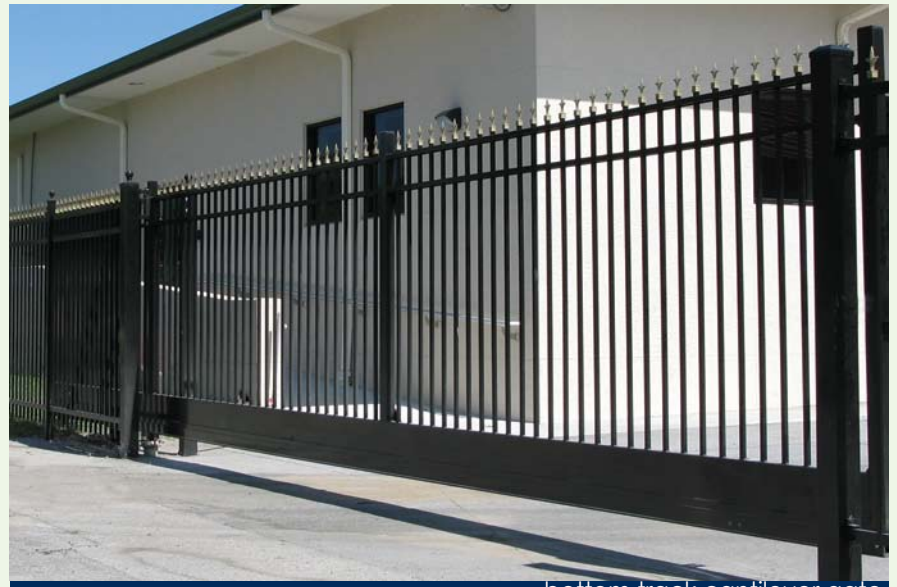
bottom track cantilever gate
